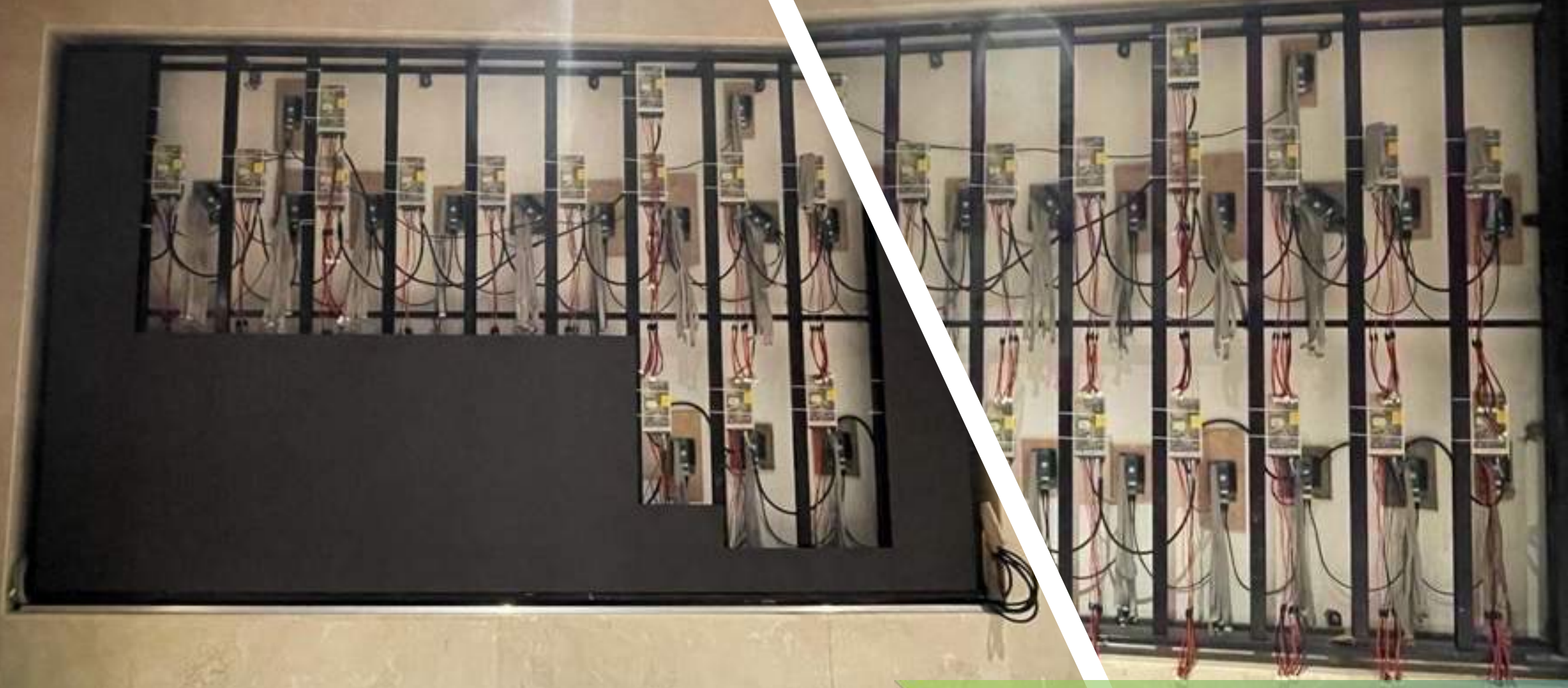
Phoenix Palladium Mall - Mumbai P2.5 wall cavity installation
